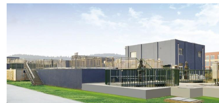
▲ World-class Advanced Sewage Treatment Station
